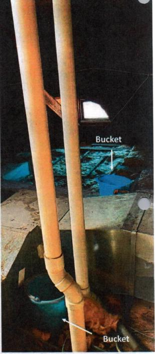
The attic is difficult to photograph on cloudy days, but these two photos demonstrate the myriad of water leaks. The photo on the left shows the attic under the center dormer on the east side. The photo on the right shows the HVAC unit near the southwest dormer.
