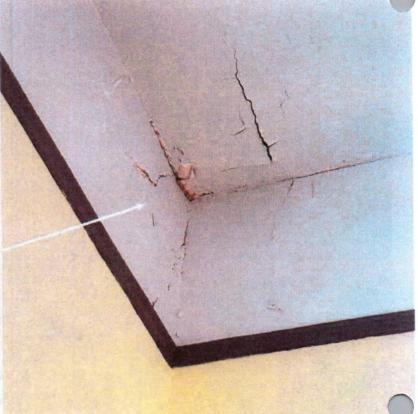
This corner leaks with nearly every rain. The damaged area on the ceiling is approximately 3 feet by 3 feet. We have taped painter's plastic to the walls to protect the woodwork. The plastic sheets drain into a plastic tub. Note the brown water in the tub. (We normally hide this behind a small folding screen.) All of the photos that were once displayed in this area have been removed to prevent damage.
